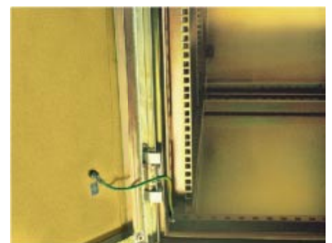
Hinge side of door showing earthing
